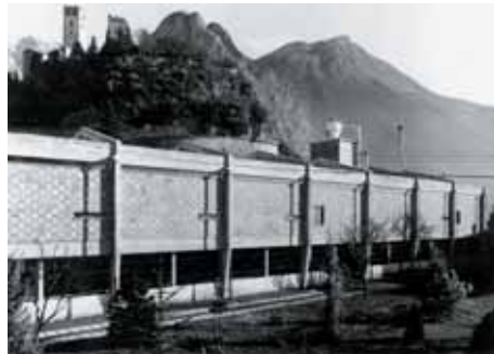
Fantoni plant, Gemona, by the architect C. Lucci.
